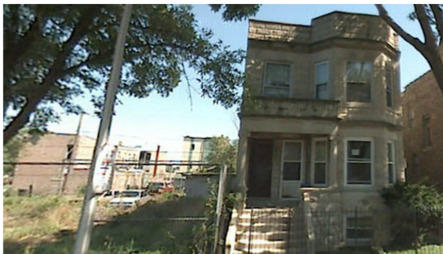
1615 South Trumbull Ave in 2007, looking like it's the next to go.
